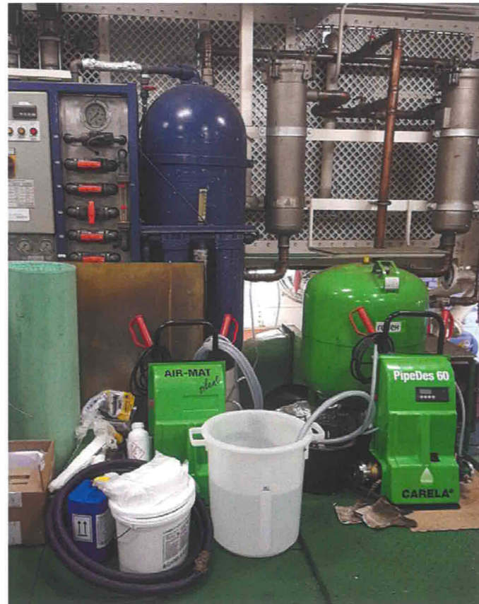
Equipment for cleaning on board
