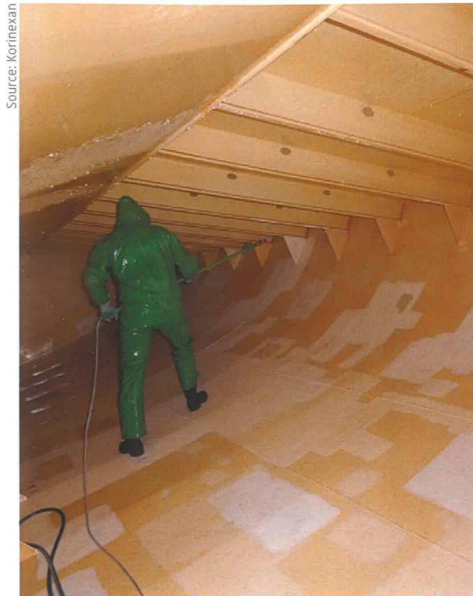
Fresh water tank during professional cleaning
